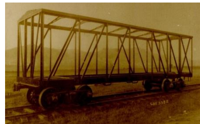
Built by ACF's Huntington Shops in 1904, these double sheathed N&W boxcars were among the first in the country built with steel body framework. ACF builder's photo, St. Louis Mercantile Library collection.
